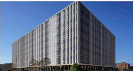
Procon provided construction management, and commissioning services for building envelope repair, systems modernization and asbestos abatement in a fully occupied 370,000 square foot office building.
